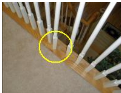
10.5 Picture 1 Railing on the 2nd floor
