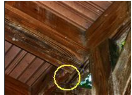
3.3 Picture 3 Deck joist at right side
