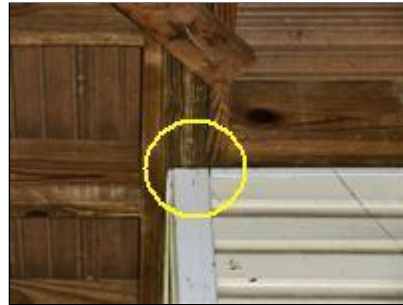
3.3 Picture 2 Deck joist at left side
